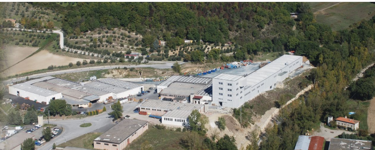
(Aerial View of Tratos Cavi S.p.A. Pieve Santo Stefano (AR) Italy)
