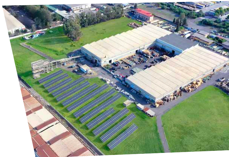
Photovoltaic panel installation at the Tratos Cavi Catania plant
