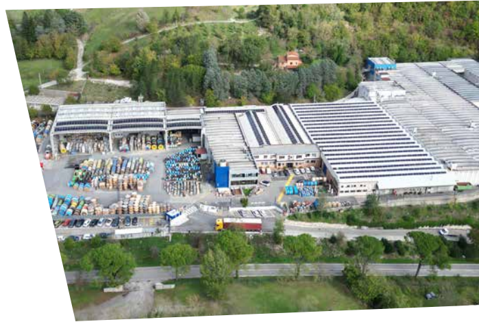
Photovoltaic panel installation at the Tratos Cavi plant in Pieve Santo Stefano
