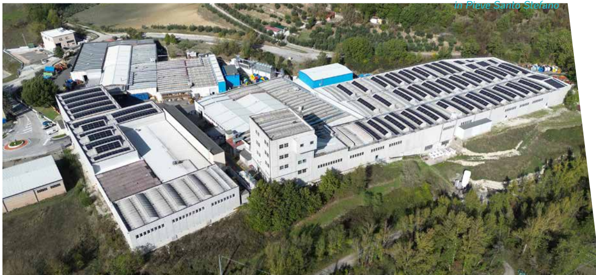
Photovoltaic panel installation at Tratos HV
