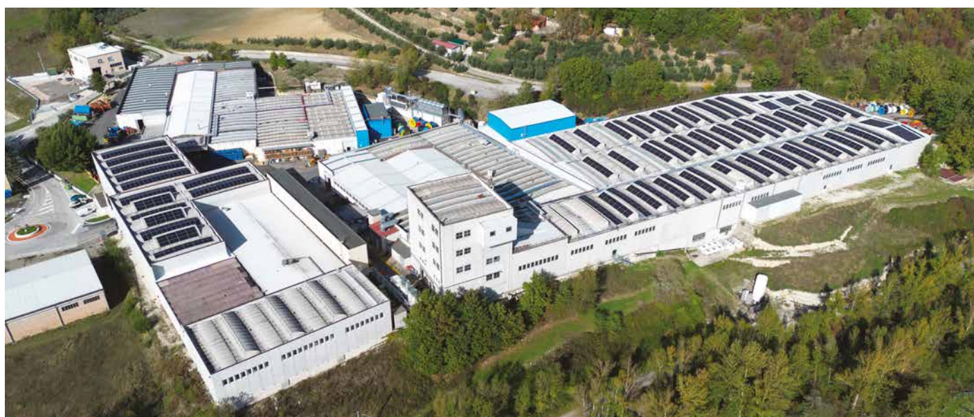
Figure 6 Installation of photovoltaic panels at Tratos HV
