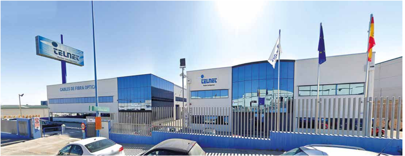
Figure 5 Telnet Fiber Optic S.L.U based in Zaragoza, Spain. Production of fibre optic cables
